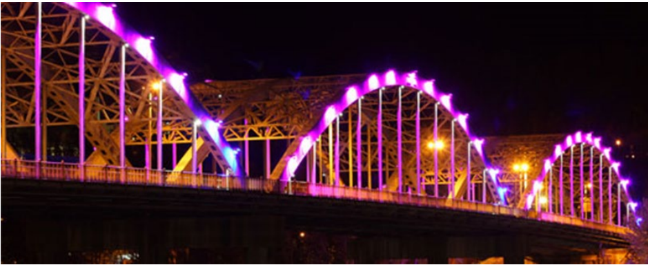
City of Trail Victoria Street Bridge $510,000
